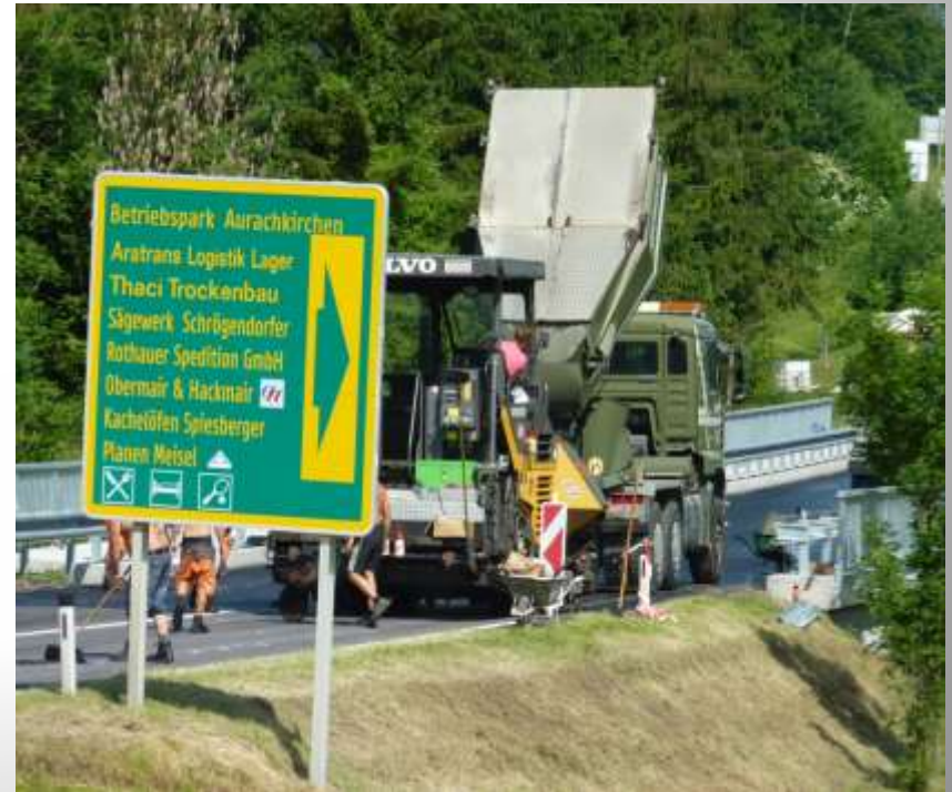
Thermal Scanner on the Paver
