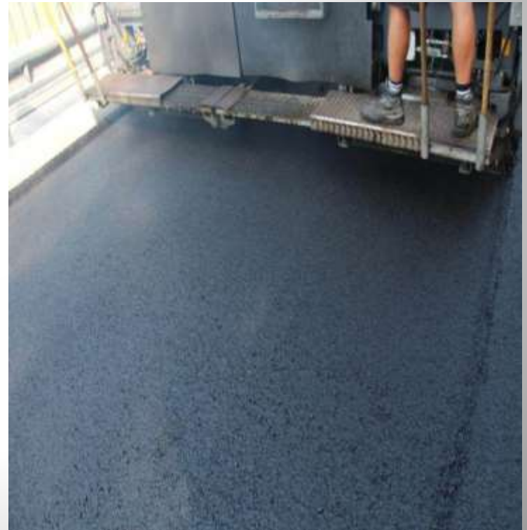
Asphalt behind the Paver
